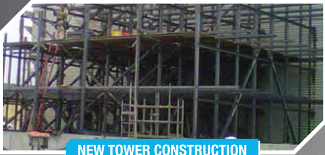
NEW TOWER CONSTRUCTION
