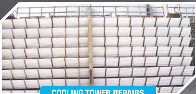
COOLING TOWER REPAIRS
